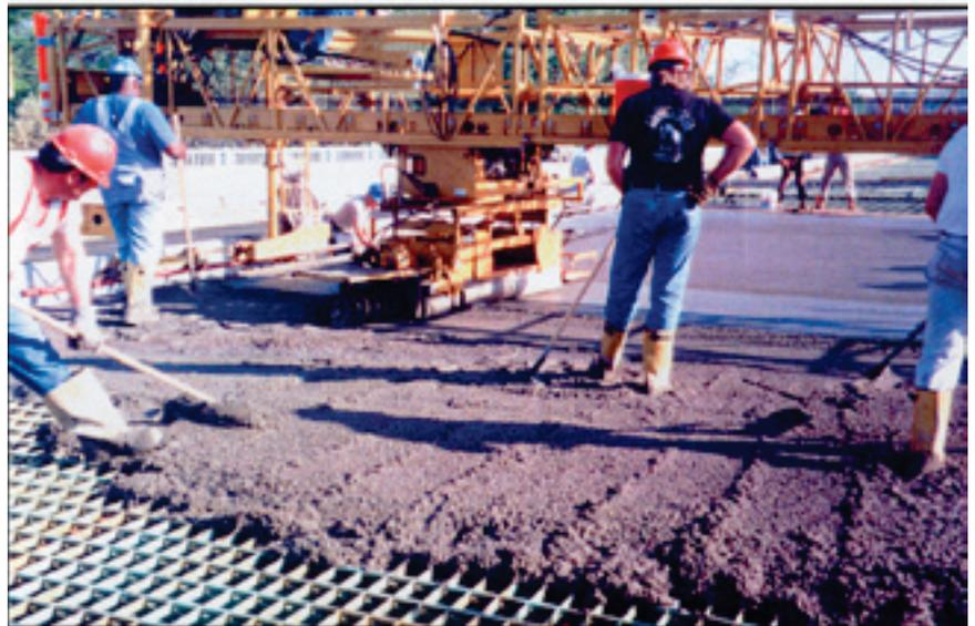
structure and provides protection to the steel grid. This protection assures that the grid, and the depth of concrete within the grid, will be structurally sound when the original overfill needs to be replaced. This scenario is illustrated quite well by the following case study of the Verrazano Narrows Bridge.
